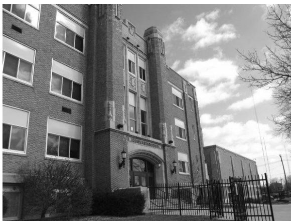
Figure 6.1: Messmer with Gym Addition. Source: Messmer High School
