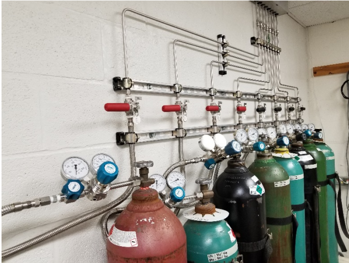
Figure 12: Fuel and Oxidizer Supply for Vitiated Heater
