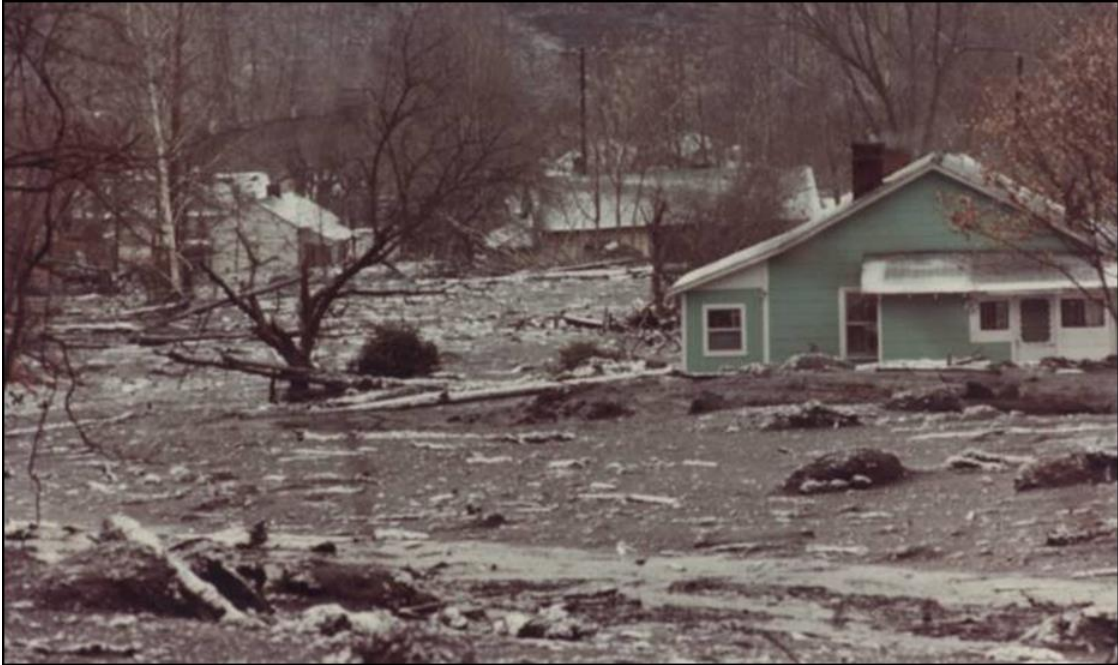
Figure 1.5: Devastation of downstream as a result of tailings slurry flow at Manalapan Mining, Brookside, Kentucky in 1980, (courtesy of Josh Phillips, 2012).
