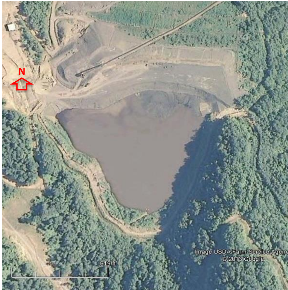
Figure 1.7: Aerial photo of Abner Fork impoundment, (Google Maps, 2013a).
