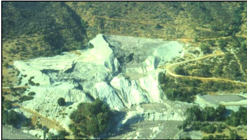
Figure 1.4: An aerial view of the 1985 Veta De Agua tailings dam failure in Chile (Castro and Troncoso, 1989).
