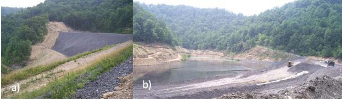
Figure 1.10: Big Branch impoundment, (a) Downstream, (b) Upstream
