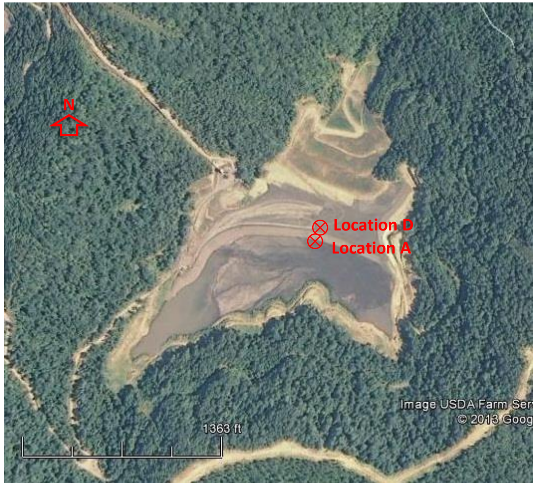
Figure 2.5: Testing and sampling locations at Big Branch impoundment, (Google Maps, 2013b).
