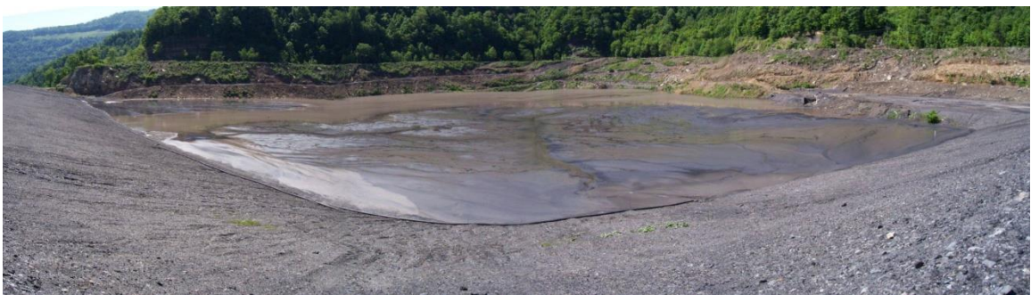
Figure 1.8: Upstream view of the Abner Fork impoundment in Harlan County, Kentucky.
