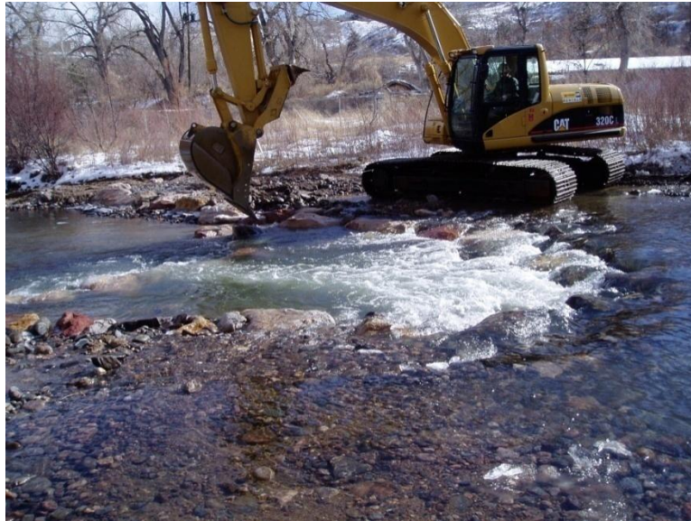
Figure 1. Photograph of a stream restoration project under construction in Clear Creek, Golden, Colorado, showing an excavator placing boulders in a gravel-bed river to control fluid and sediment transport mechanics in order to promote stable fisheries and channel stability
