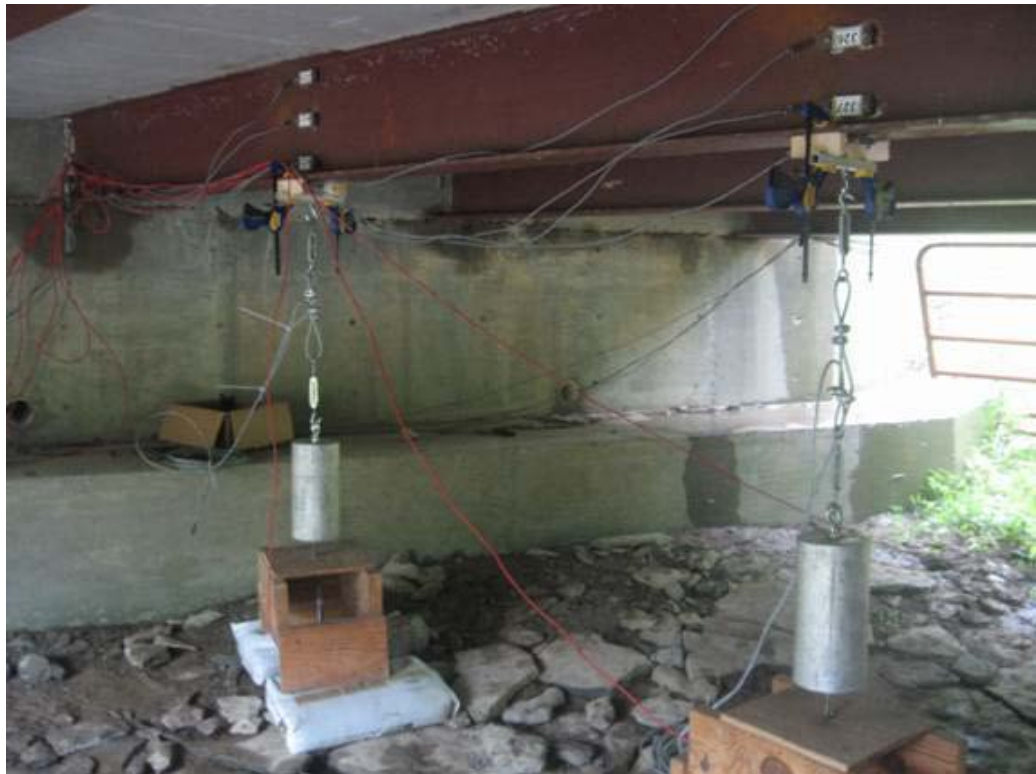
Fig. 5.25: Wire mounted weights hung above LVDT locations on girder G3
