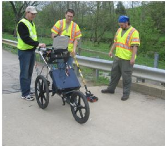
(a) Locating rebar positions on the top surface
