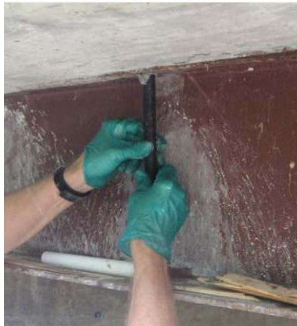
Fig. 5.10: Inserting threaded rod with twisting motion
