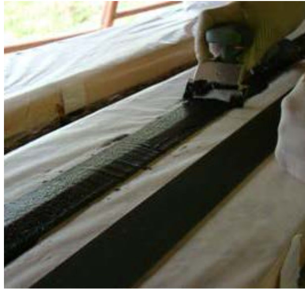
Fig. 5.19: Spreading of epoxy with V-notch trowel
