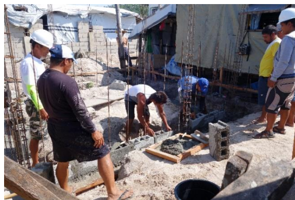
Demonstration training for block laying.
