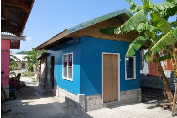
Alternative timber design house with masonry skirt.
