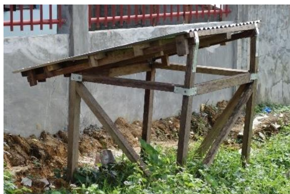
Scale model used to demonstration key messages for safer building construction.
