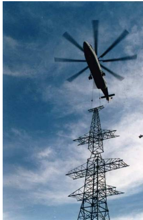
Figure 3: Helicopter carrying a power transmission tower 3 .
