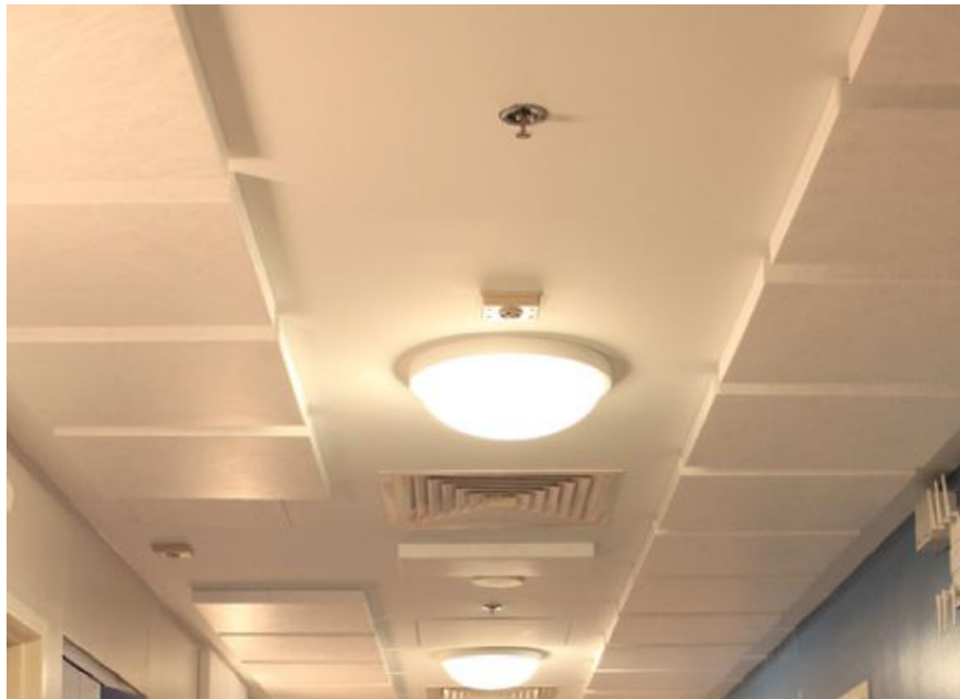
Figure 27. Installed Panels in Weinberg 5A
