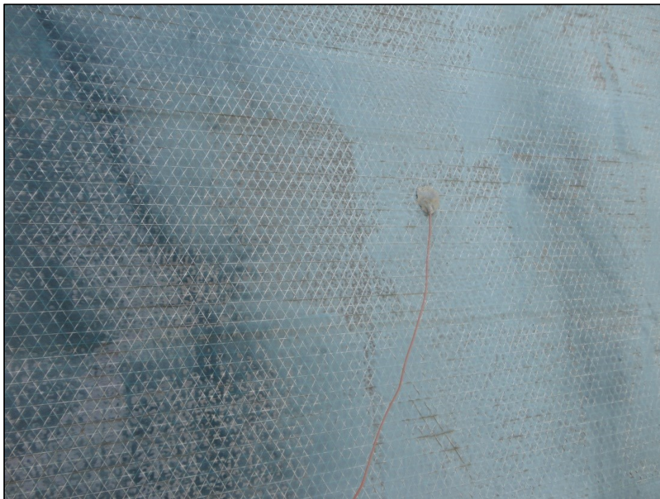
Figure A18: Photo at Location 5 (North Side of Wall 2)
