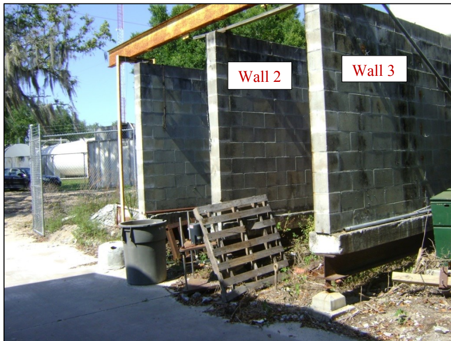
Figure 17: Overhanging End of Walls
