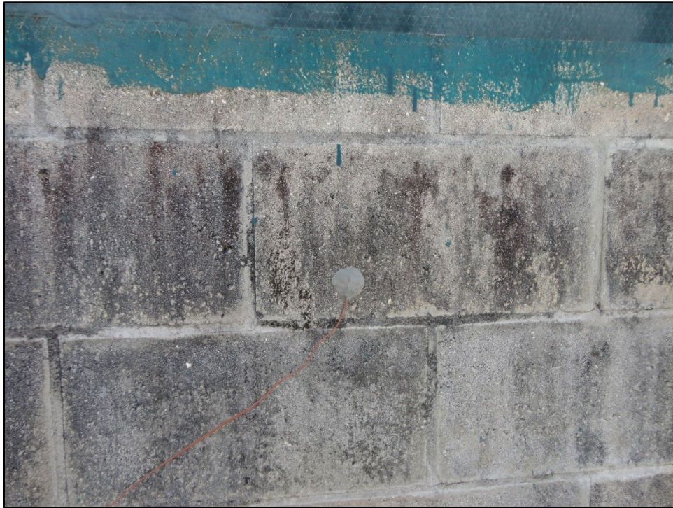
Figure A75: Photo at Location 24 (North Side of Wall 2)
