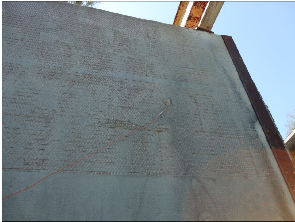
Figure A27: Photo at Location 8 (North Side of Wall 2)
