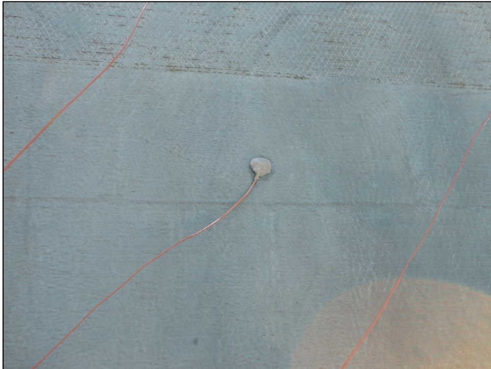
Figure A45: Photo at Location 14 (North Side of Wall 2)
