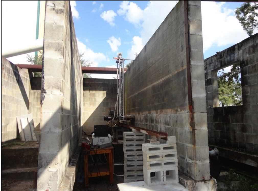
Figure 49: Thermal Scanner Setup on Wall 3
