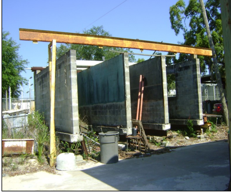
Figure 2: Photograph of Masonry Walls at USF
