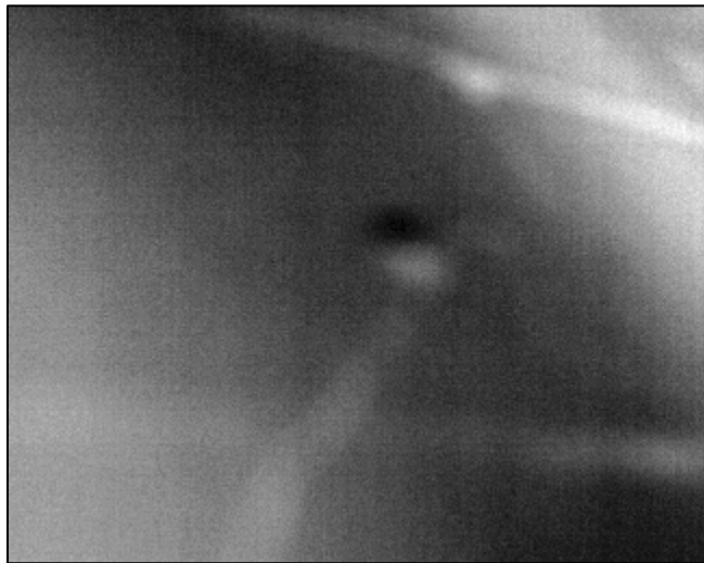
Figure A40: Thermal Image at Location 13 at 1:02 PM (North Side of Wall 2)
