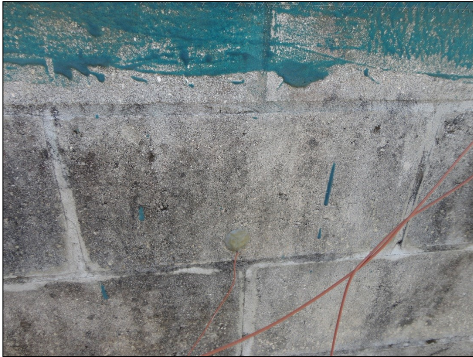
Figure A63: Photo at Location 20 (North Side of Wall 2)
