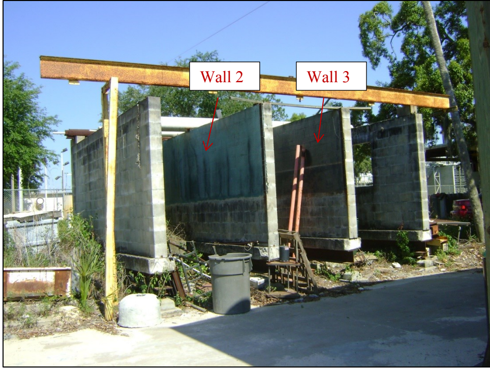
Figure 64: The Two Walls Investigated
