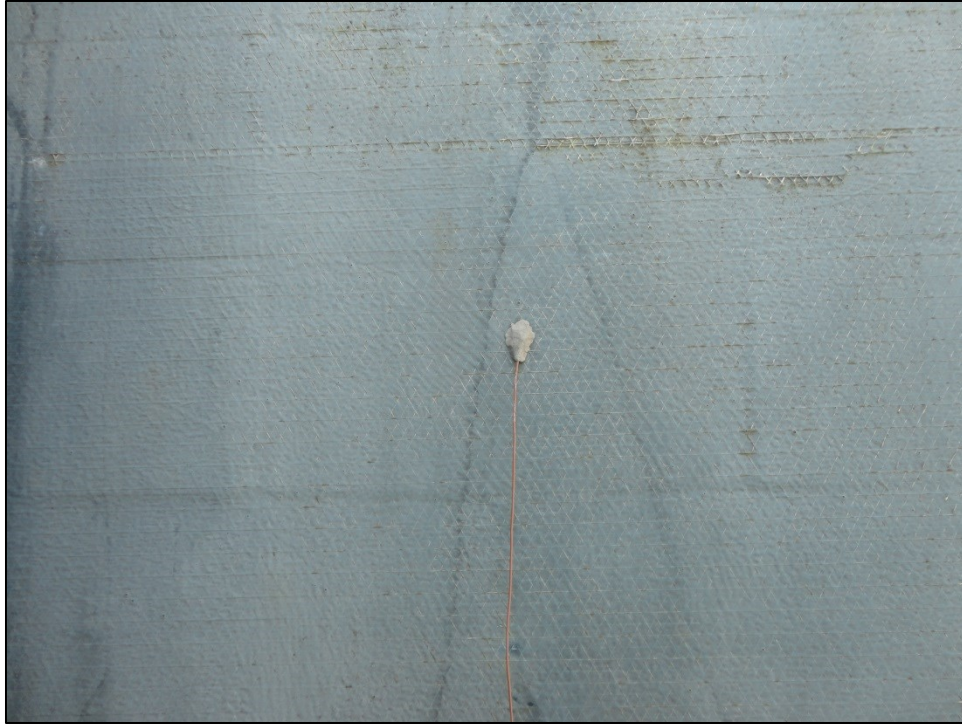
Figure 32: Wall 2 Location 2 Photo (North Side)
