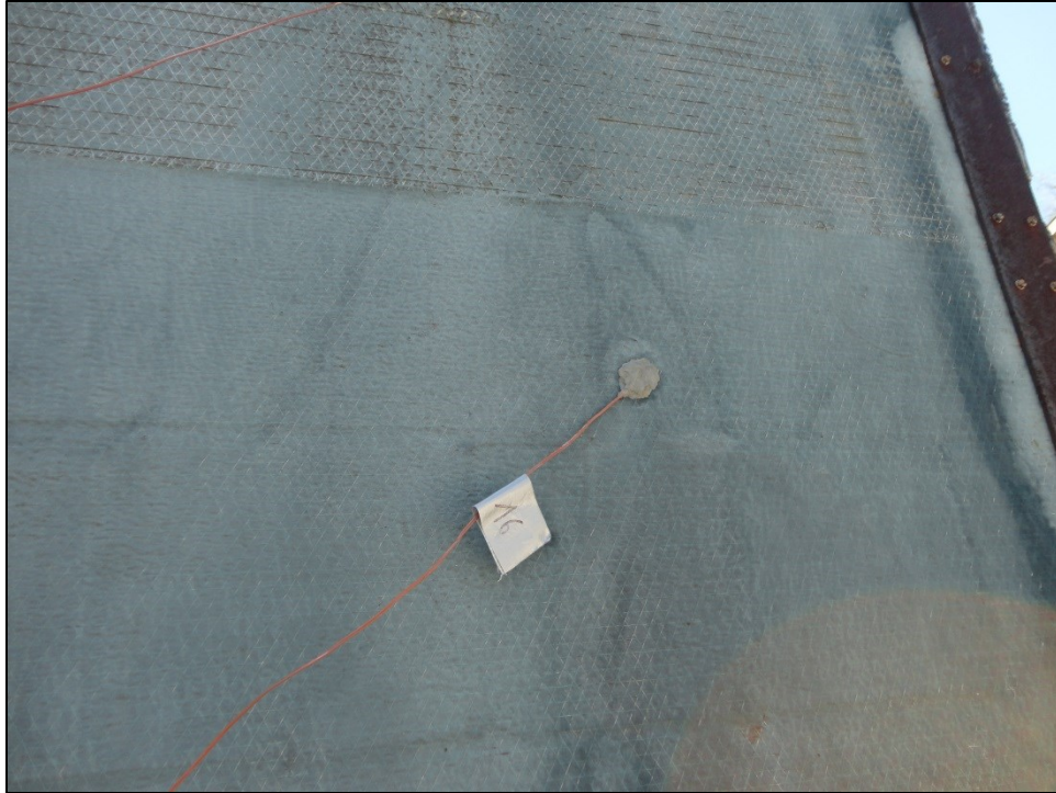
Figure 38: Location 16 Photo (North Side of Wall 2)
