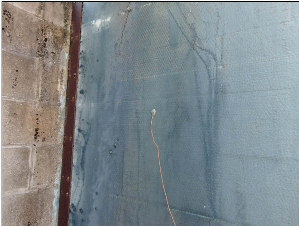
Figure A6: Photo at Location 1 (North Side of Wall 2)
