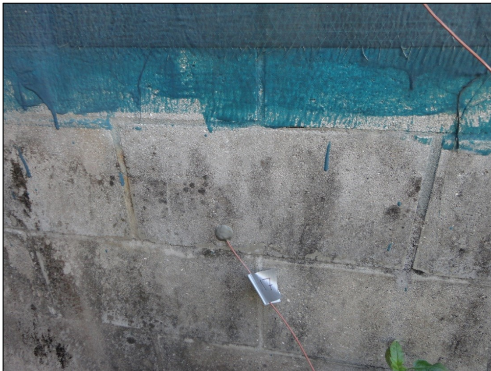
Figure A54: Photo at Location 17 (North Side of Wall 2)
