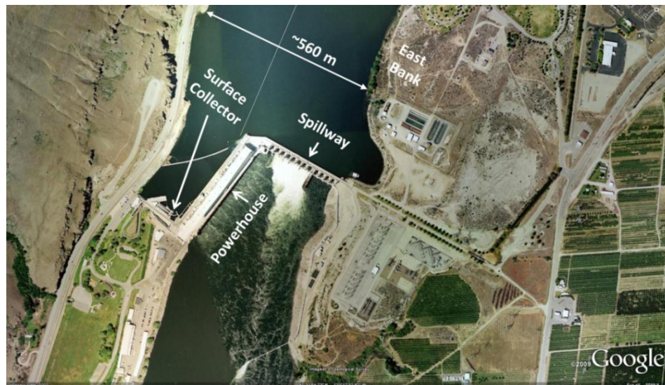
Figure 3.1 Dam 1 aerial photo.
