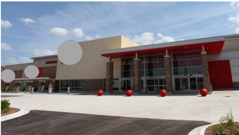
Figure 4: The case study building upon construction completion.
