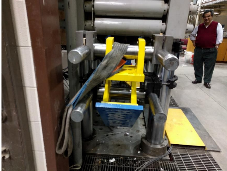
Figure 13 – With reaction bars in place, rod clamps and clevis brackets are installed.
