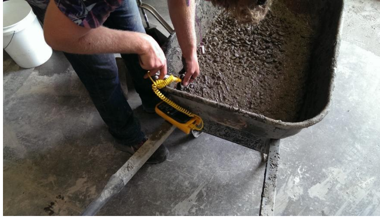
Figure 79 - Placing temperature probe
