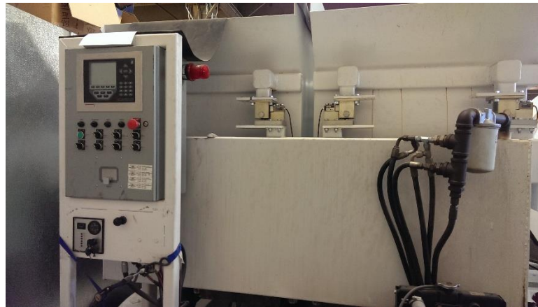
Figure 29 - Close view of mobile batch plant at Fall Line. Note load cells for weighing hopper contents.
