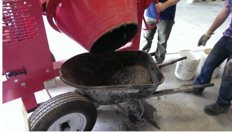
Figure 78 - Discharging freshly-mixed concrete
