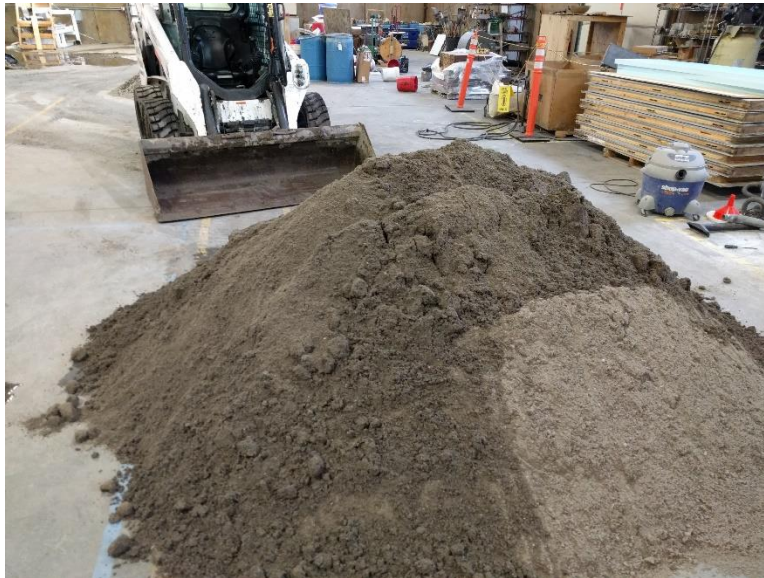
Figure 31 - Mixing fine aggregate and forming into pile.
