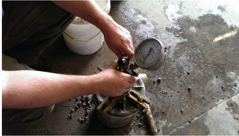
Figure 85 - The top portion of the air meter is installed.
