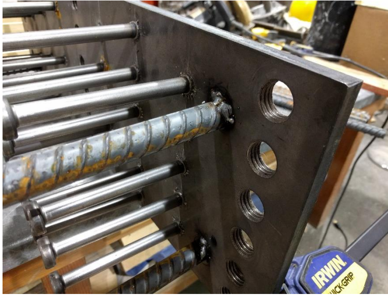
Figure 25 - MIG-welded joint between #6 rebar and sample end plates.
