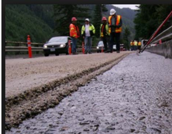
Figure-37 Final product installed
