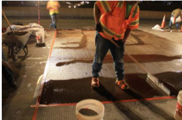
Figure-34 Surface preparation & resin application
