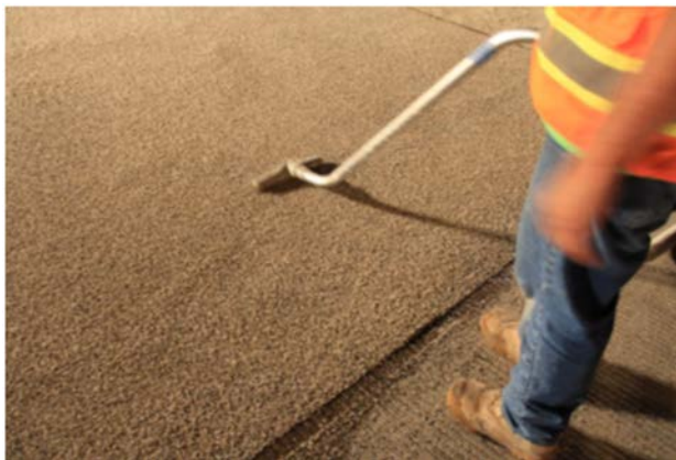
Figure-36 Removal of excess material
