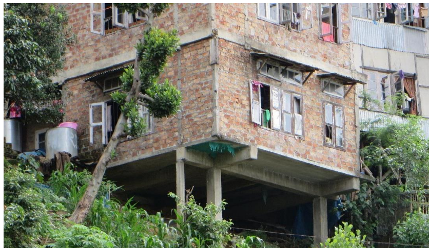
Figure 4. Typical residential building in Aizawl with reinforced concrete frame and masonry infill.
