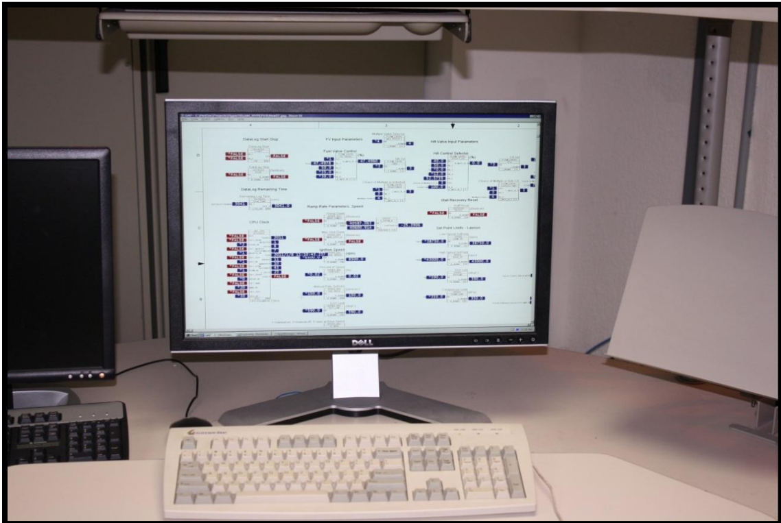
Figure 3.7: AtlasPC control system computer
