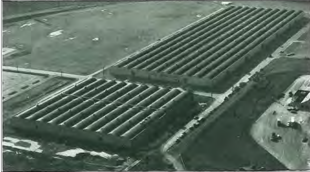
Figure 5.1: Pennsylvania Warehouse Complex, (Billington, 1965)
