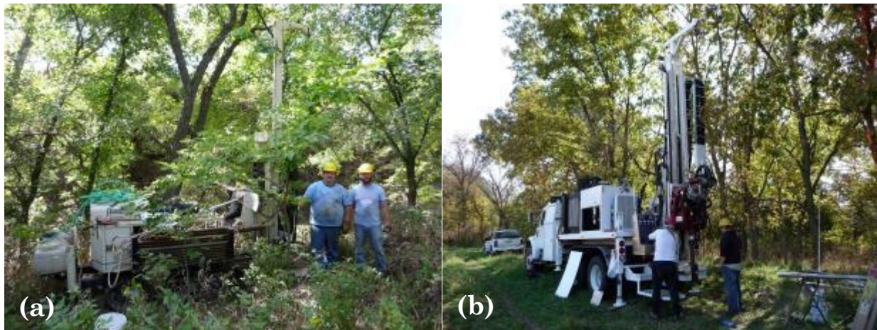
Figure 3. 3. (a) Dual-rod Geoprobe direct push system that was used in drilling the deep alluvium wells (KGS, Ed Robelet and Steve from right to left). (b) RotoSonic drill rig that was used to make the bedrock well.
