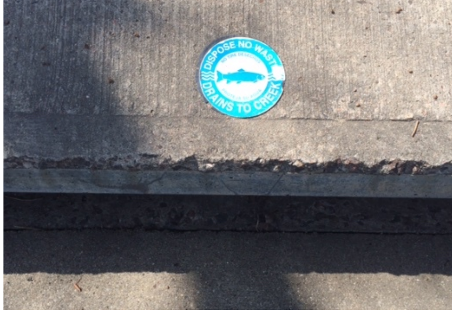
Figure 1-2: Storm Drain "Dispose No Waste - Drains to Creek", Boulder, Colorado (Photo by Mary Jean O'Hair)
