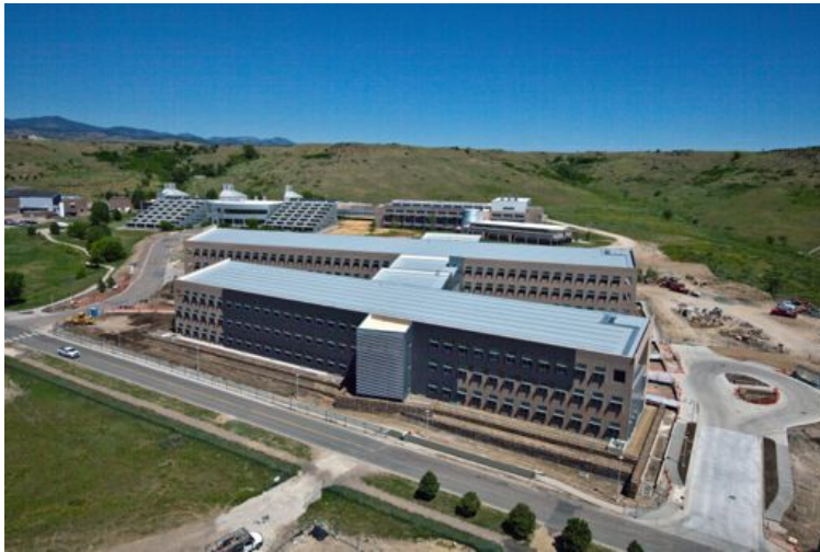
Figure 5.3: Research Support Facility (RSF) building in Golden, Colorado.
