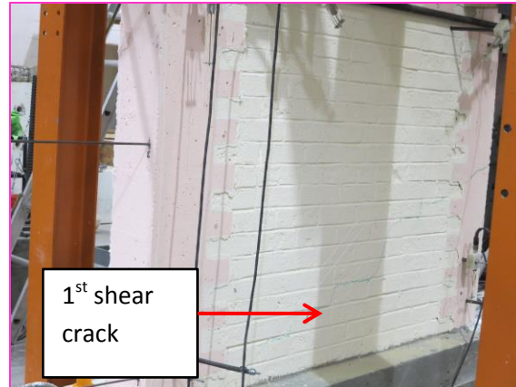
Figure 3-42. Nguyen CM Wall 1 1 st shear crack
