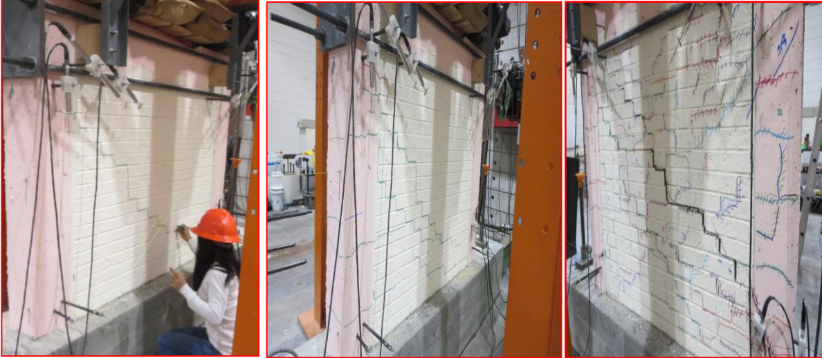
Figure 3-48. Nguyen CM Wall 2 shear cracks
