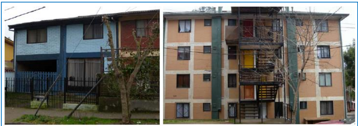
Figure 2-5. Typical Confined Masonry Buildings in Chile (left: 2 story apartment, right: 4 story apartment) (Brzev et al., 2010)
