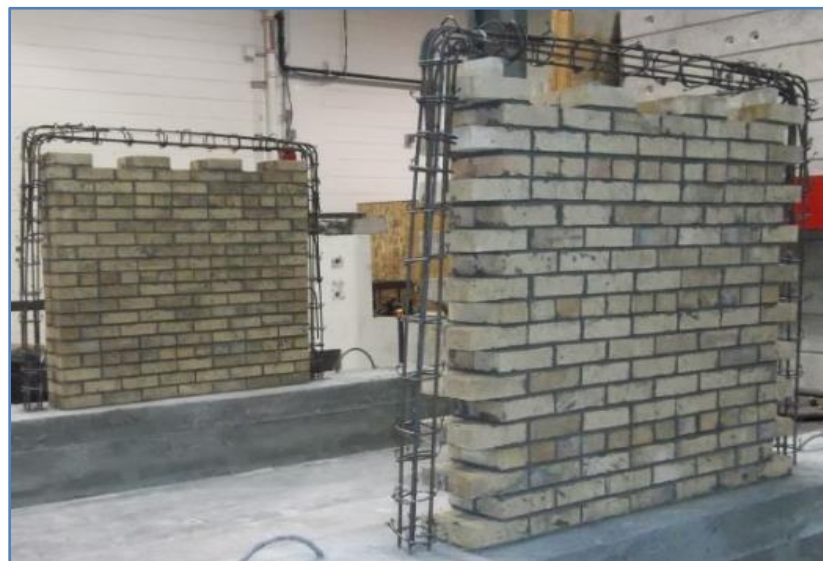
Figure 3-11. Construction of masonry wall panels
