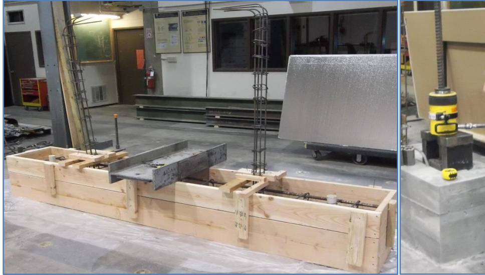
Figure 3-3. Footing and reinforcement for tie elements; Post tension jack on Dywidag rod
