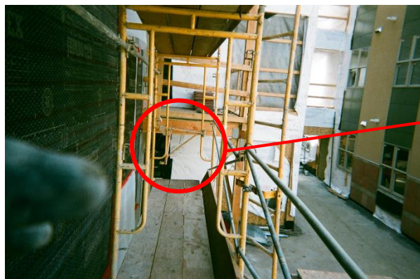
Figure 4.3: Scaffold Railing Proper
