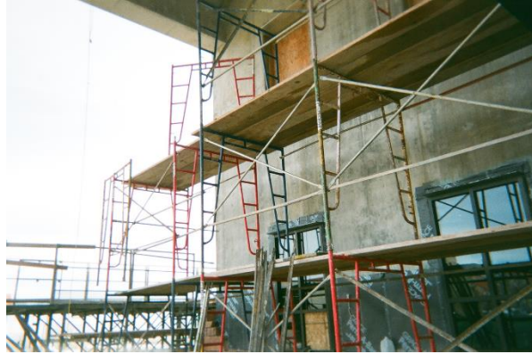
Figure 4.12: Hispanic Crew and Scaffold
