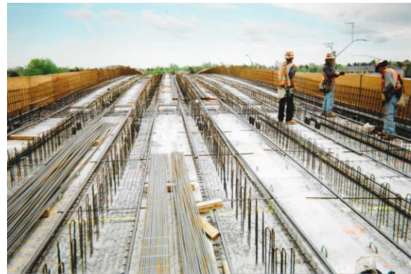
Figure 4.9: Rebar Final Placement Location
