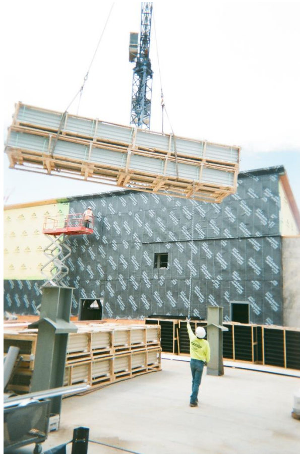
Figure 4.16: Spanish Speaking Worker Helping with Crane
