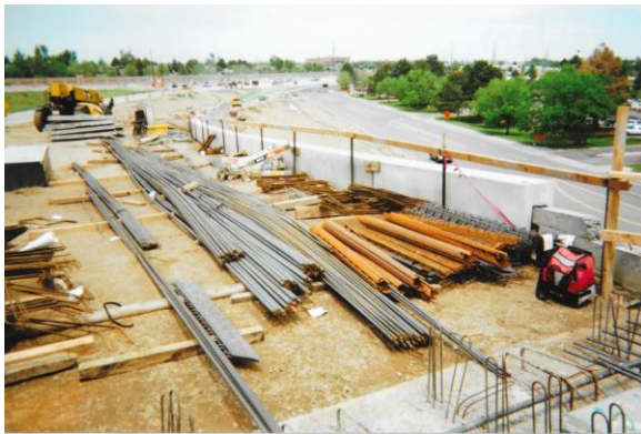
Figure 4.8: Rebar Storage Area
