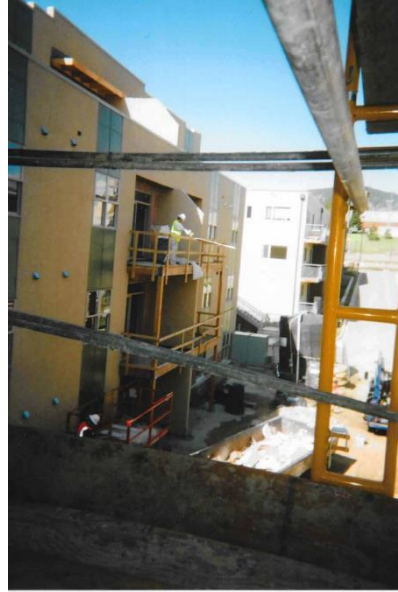
Figure 4.17: Worker Throwing Debris
