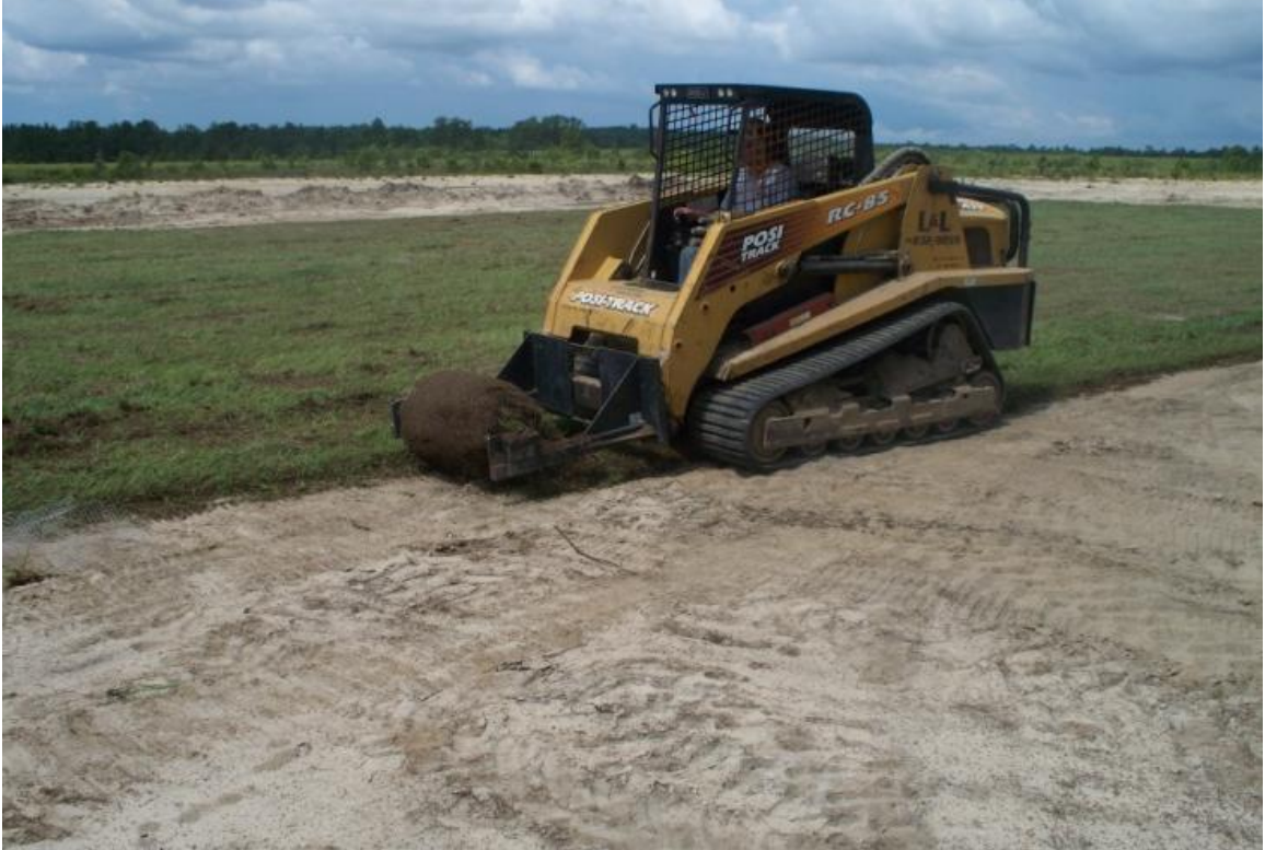
Figure A-2. Installation of Bahiagrass Pensacola sod on May 26, 2009.
