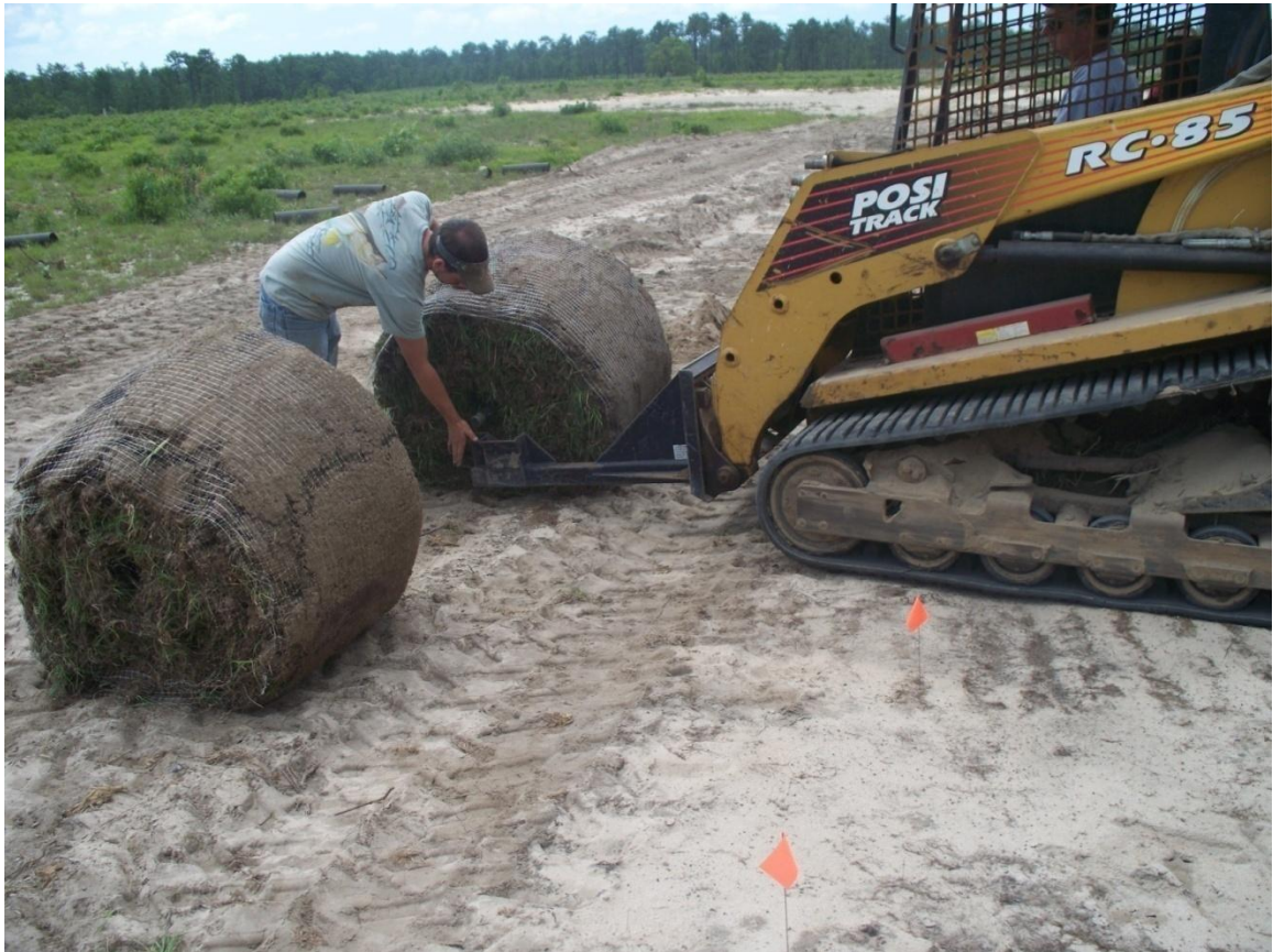
Figure A-1. Installation of Bahiagrass Pensacola sod on May 26, 2009.
