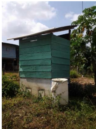
Figure 8. Double-Vault Urine-Diverting Composting Latrine in the Comarca Emberá-Wounaan (Courtesy of Daniele Renzi)
