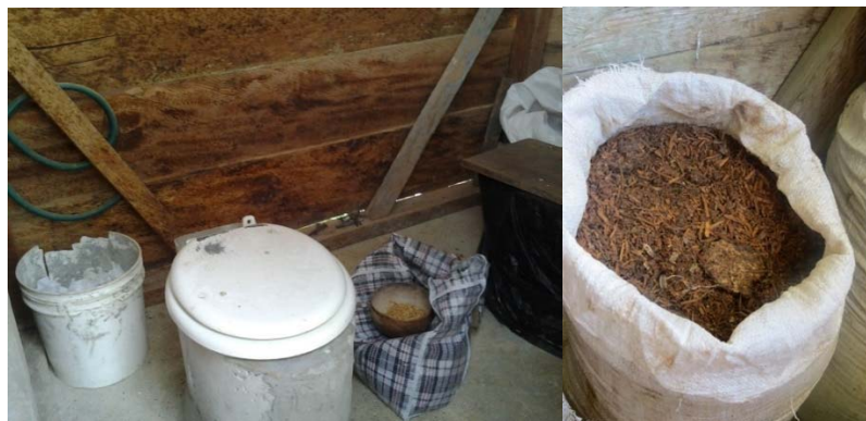
Figure 10. Examples of Desiccant Stored Next to Toilet for Application after Defecation (Courtesy of Danielle Renzi and Patricia Wilbur)
