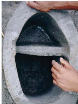
Figure 6. Aerial View of Composting Latrine Toilet Seat with Separation for Urine and Feces (Peace Corps Panama, 2010).
