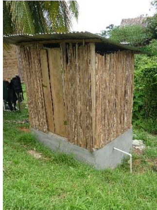
Figure 9. Double-Vault Urine-Diversion Composting Latrine in a Ngäbe Community in Bocas del Toro Province (Courtesy of Author)
