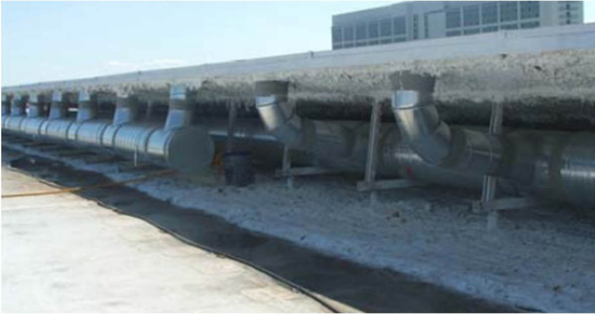
Figure 3.4: PV/T Array After Duct and Insulation Installation (rear)
