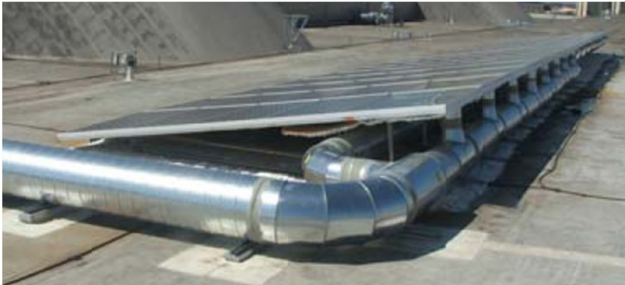
Figure 3.3: PV/T Array After Duct and Insulation Installation (side)
