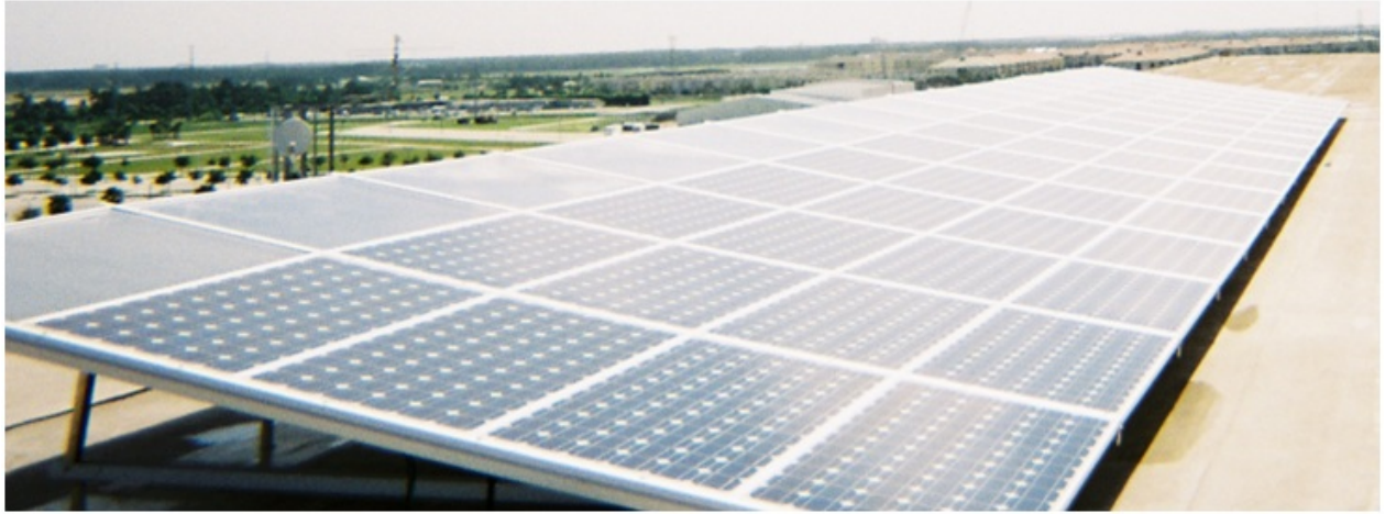
Figure 3.2: PV/T Array Before Duct Installation
