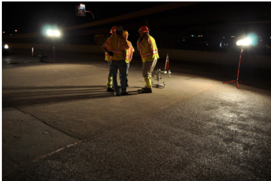
Figure 4-15 Installation Debriefing and Clean-up (3:30 AM)
