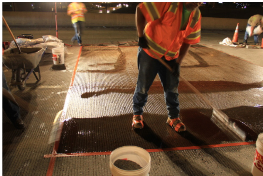
Figure 4-7 Application of First Layer (11:15 PM)
