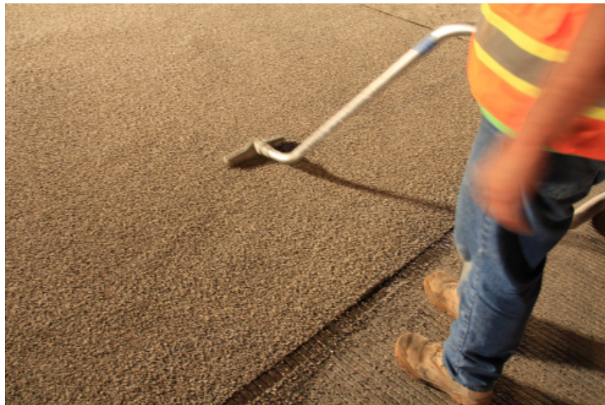
Figure 4-11 Removal of Loose Aggregate (12:30 AM)
