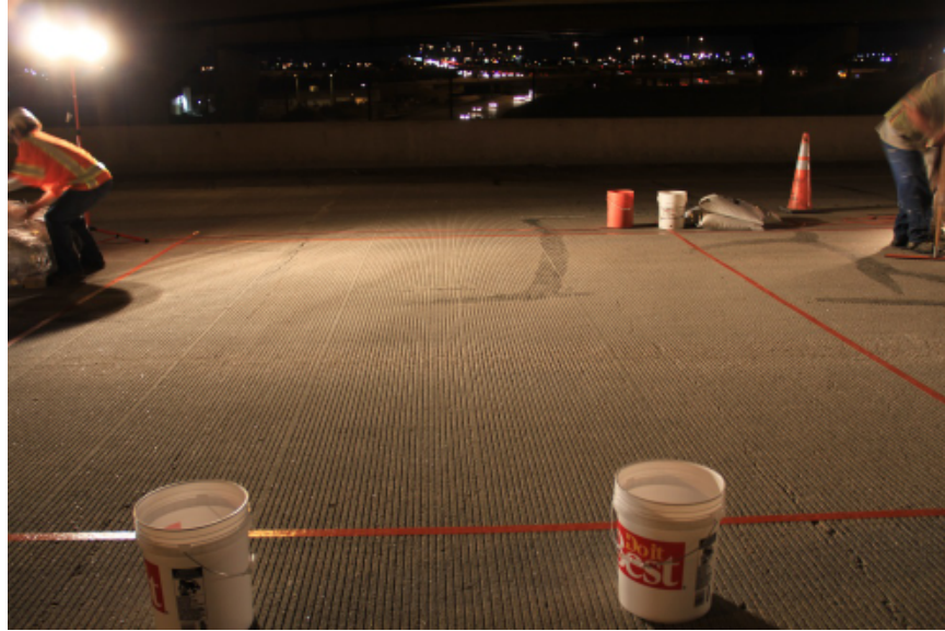
Figure 4-4 Prepared Surface (11:00 PM)
