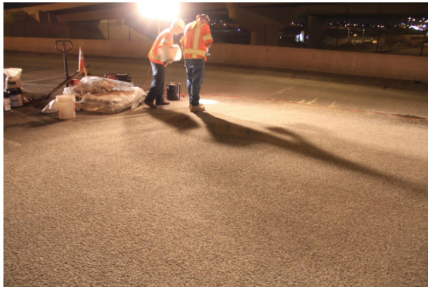
Figure 4-13 Repeat Aggregate Broadcasting/Curing/Removal (2:00 AM)
