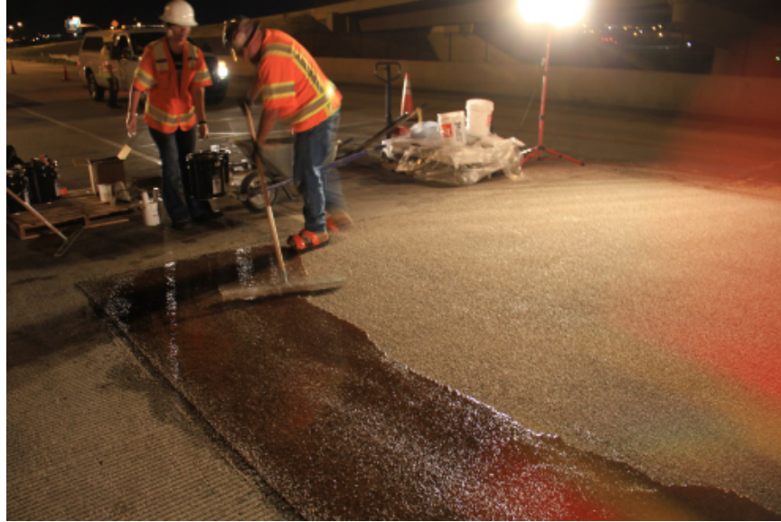
Figure 4-12 Application of 2nd Coat (1:00 AM)
