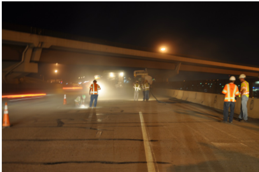
Figure 4-3 Shotblasting (10:30 PM)
