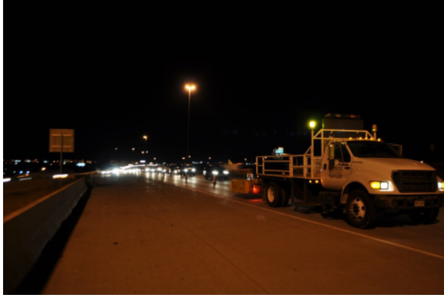
Figure 4-2 Traffic Safety Set-up (10:00 PM)
