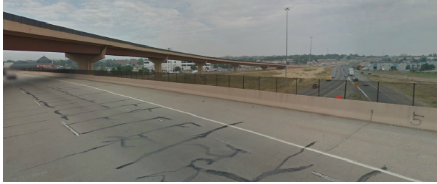
Figure 1-1 Deck Surface Prior to Installation
