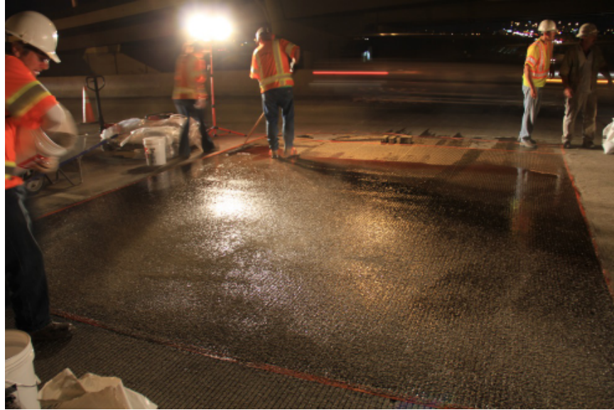
Figure 4-8 Broadcasting Aggregate (11:15 PM)
