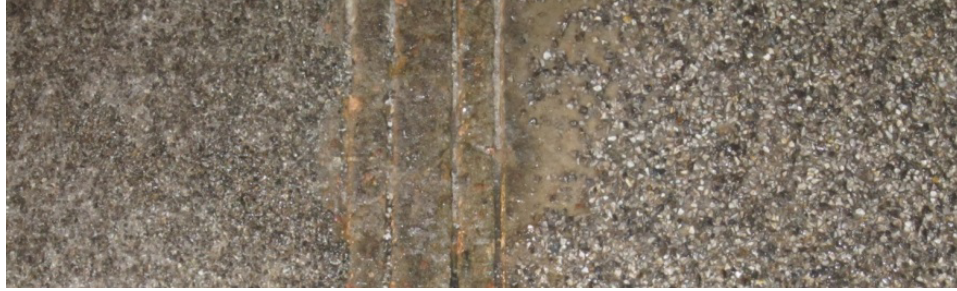
Figure 5-28 Joint between Epoxy and MMA sections
