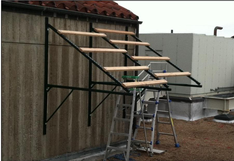
Figure 40. Photo of the frame structure. Support for the plywood is 2x4's spaced every 24" on center. This photo is missing the cross bracing that is currently installed between the horizontal members.
