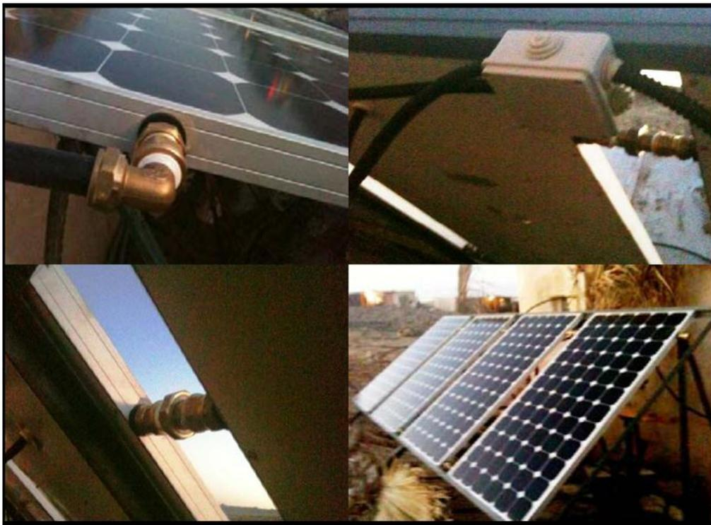
Figure 5. These photos demonstrate the concept of the PV/T designs by Millennium Solar. You can see the plumbing for the thermal component in the left-side photos. There is no building integration design or emphasis put on the aesthetics on a residence. (MillenniumSolar, 2011)
