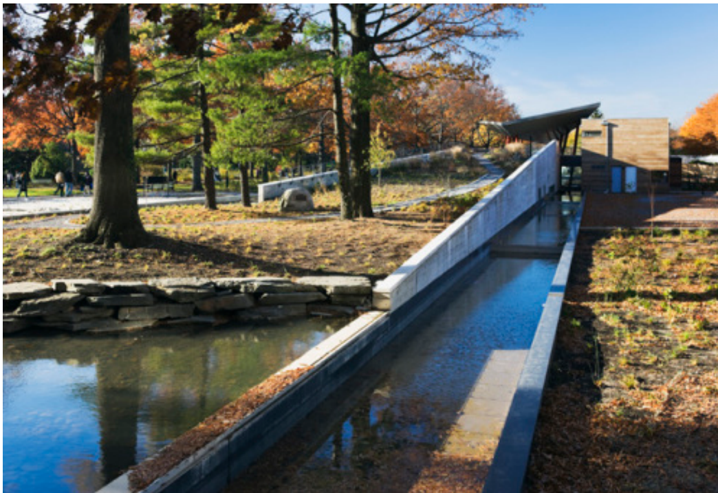
Figure 6.8: Auditorium Vegetated Roof and Separating Water Channel – Queens Botanical Garden Visitor Center
