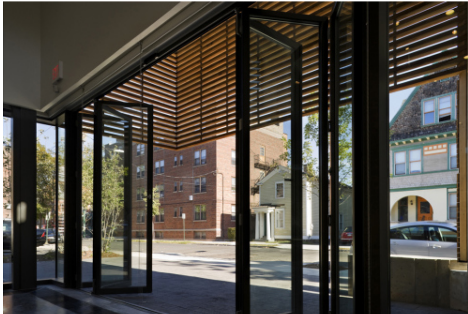
Figure 6.13: Large Opening Doors for Gallery Entry – Yale Sculpture Building and Gallery
