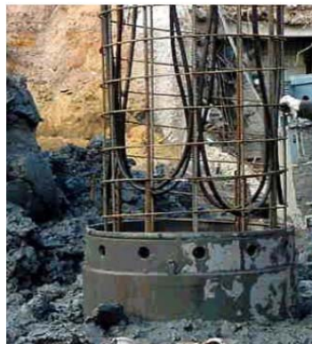
Figure 2.1: Photograph of U-tube heat exchangers attached to the reinforcement cage of a drilled-shaft energy foundation
