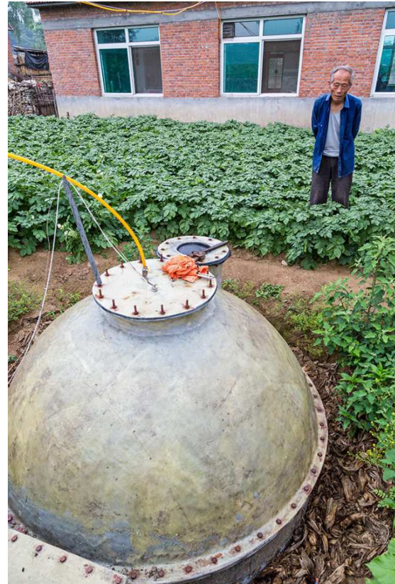
Figure 76 - A biogas reactor at a farm near Dandong, China
