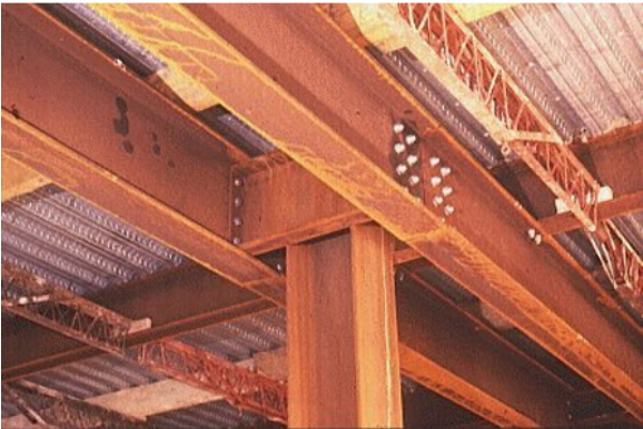
Figure 2: Web Splice (Corus Construction n.d.) & (Kulak 1975)
