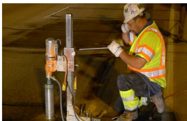
Figure 6.15 Taking cores from bridge decks
