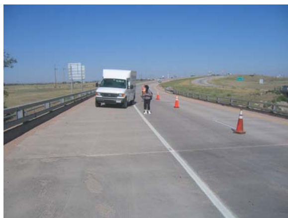
Figure 5.3 CDOT traffic control (Bridge G-22-BG)
