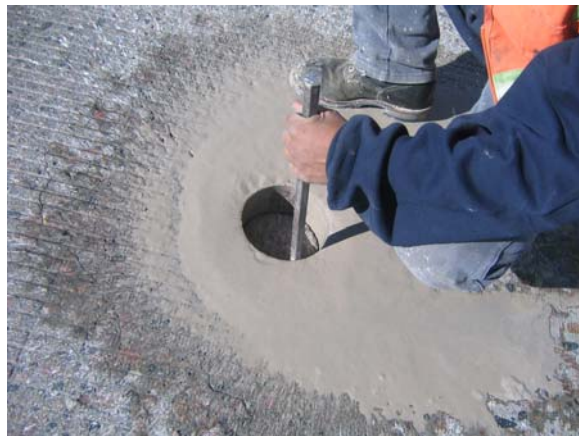
Figure 5.2 Coring concrete samples (Bridge G-22-BJ)
