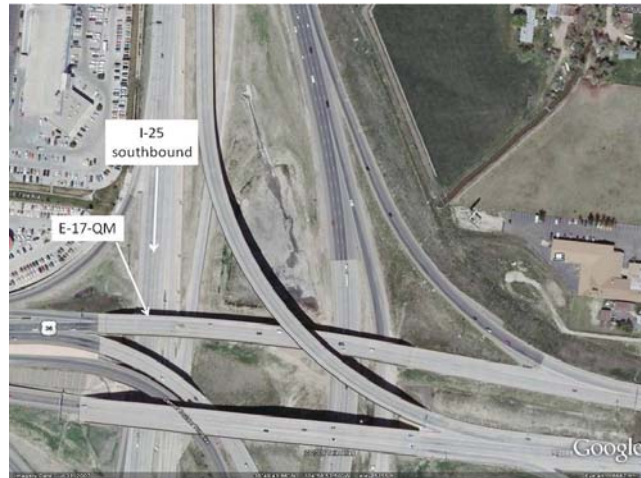
Figure 6.1 Bird's eye view on Bridge E-17-QM
