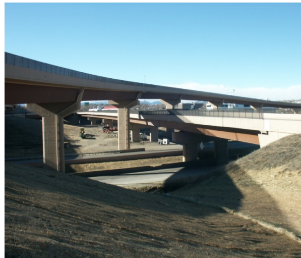
Figure 6.2 Side view of this bridge structure
