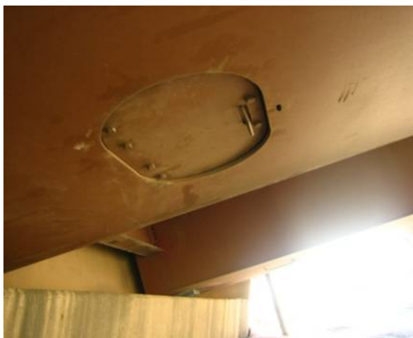
Figure 6.4 A hatch beneath the bridge for passing through
