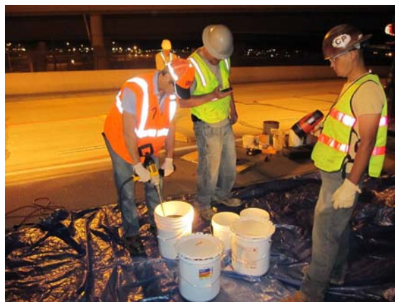
Figure 6.6 Mix chemical solutions
