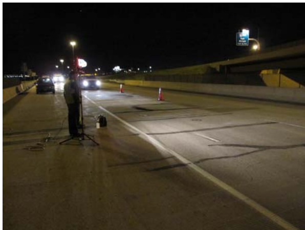
Figure 6.3 Two traffic and one shoulder lanes of the bridge
