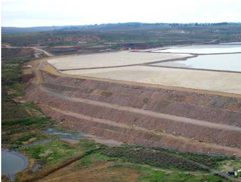
Figure 1.0.1 – shows a containment facility for tailings from a gold mine (Orosur Mining 2011)
