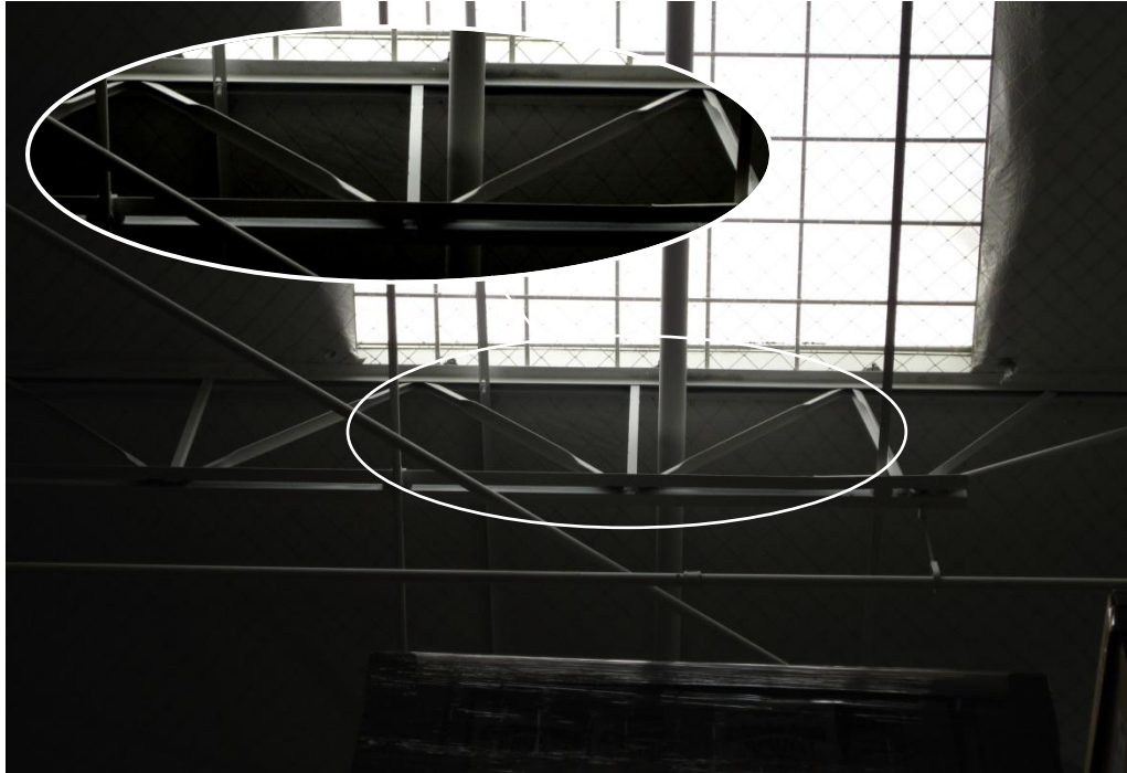
Figure 4.20 – Open web steel joist consisting of double angled chord members and crimped single angled web members with vertical elements (Building 6).
