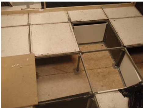
Figure 3–15: Raised Floor Plenum Partition Construction
