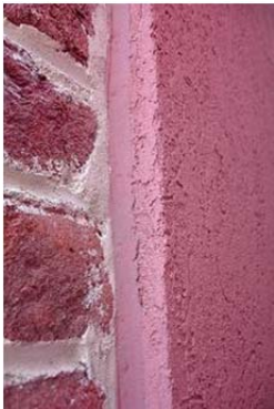
Figure 6-13: Exterior wall board insulation (CommonWealth LLC, 2009)
