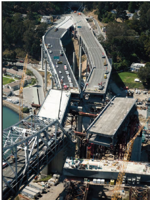
Figure 3.4 – Bay Bridge East Span Construction (TBPOC, 2010)
