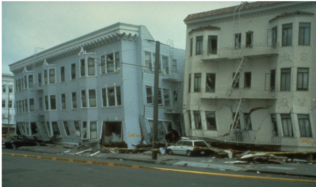
Figure 4.1 - Two multi-unit, wood-frame soft-story buildings that collapsed in the Marina District during the 1989 Loma Prieta earthquake. (ATC, 2009: Image courtesy of the National Information Service for Earthquake Engineering, University of California, Berkeley)
