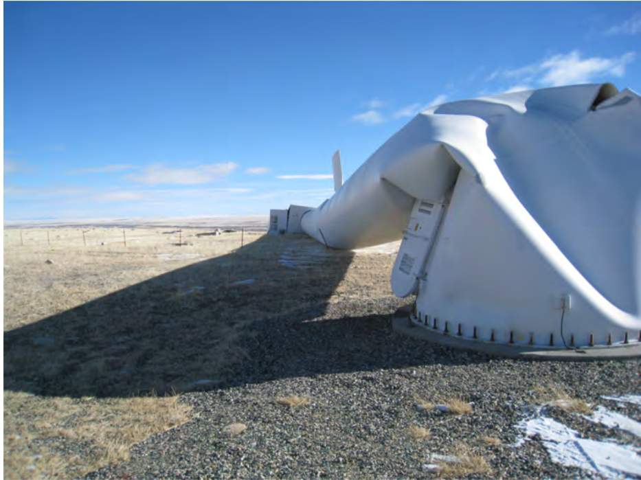
Figure 1.1: Wind turbine in Wyoming that failed due to wind loading [1]
