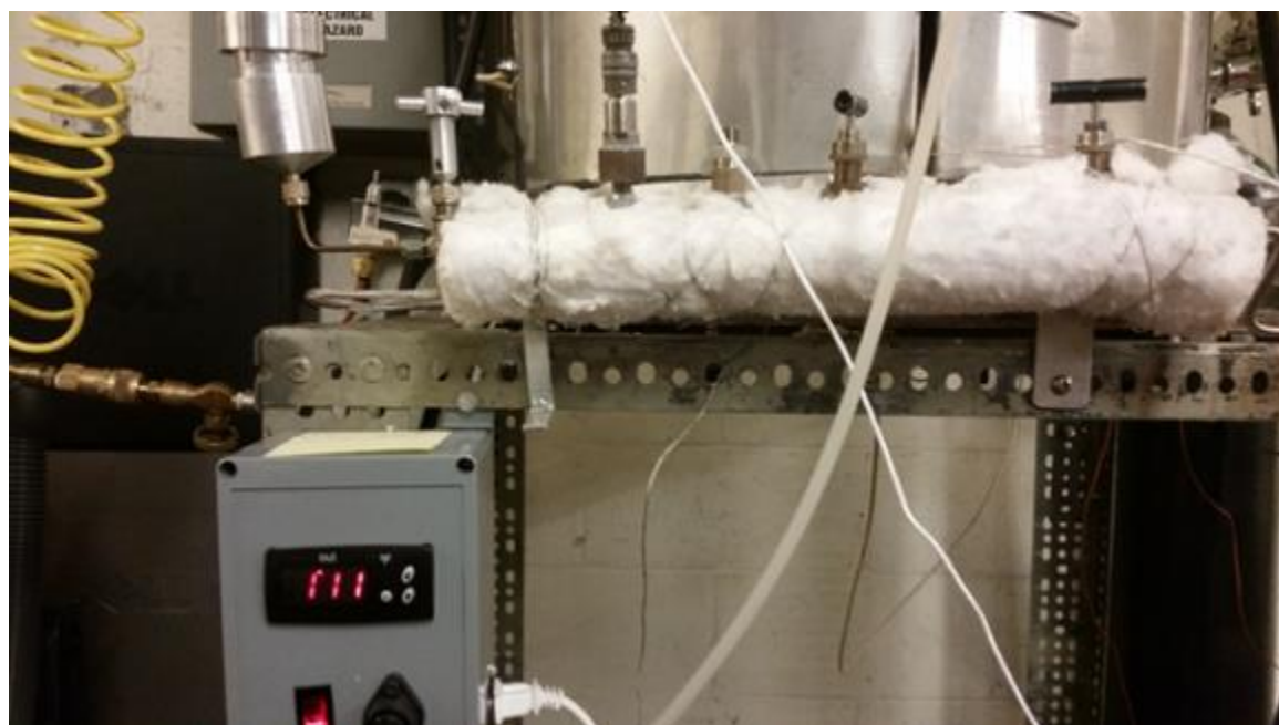
Figure 17: Heated liquid filling lines and controller
