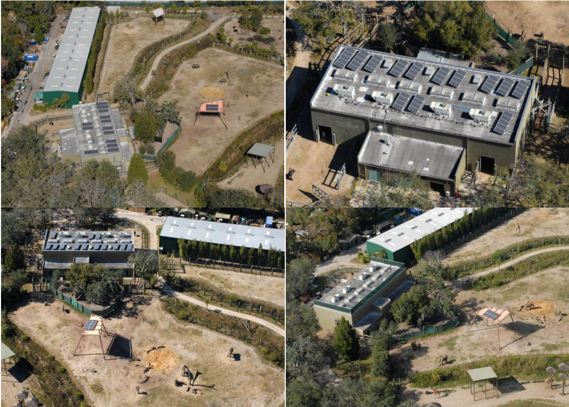
Fig. A.1 Picture of PV installation at TLPZ
