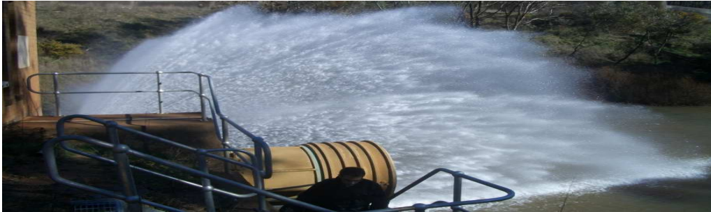
Figure 1.3: Top: Picture of a fixed-cone valve. Bottom: Picture of water release from Lake Nillahcootie.
