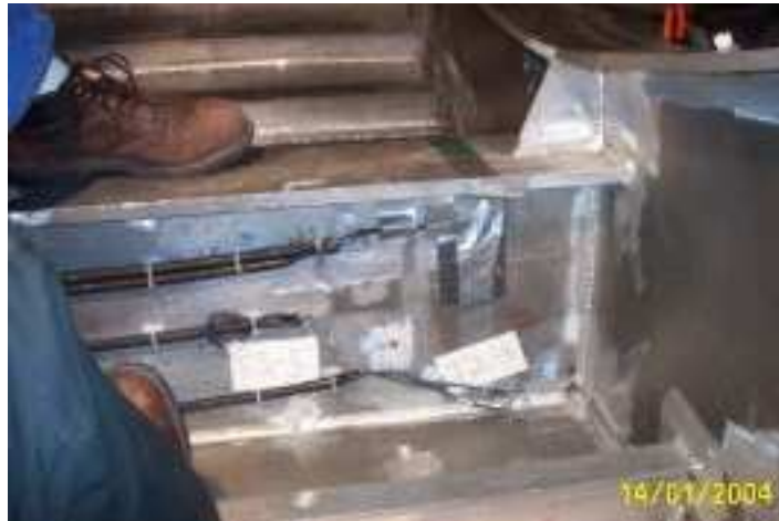
Figure 4: Installation of two sensors (T1 and T2) at frame location 26 [1]
