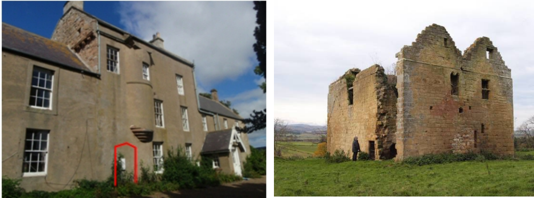
Figure 3.13. Alterations to roofs and stairs.
