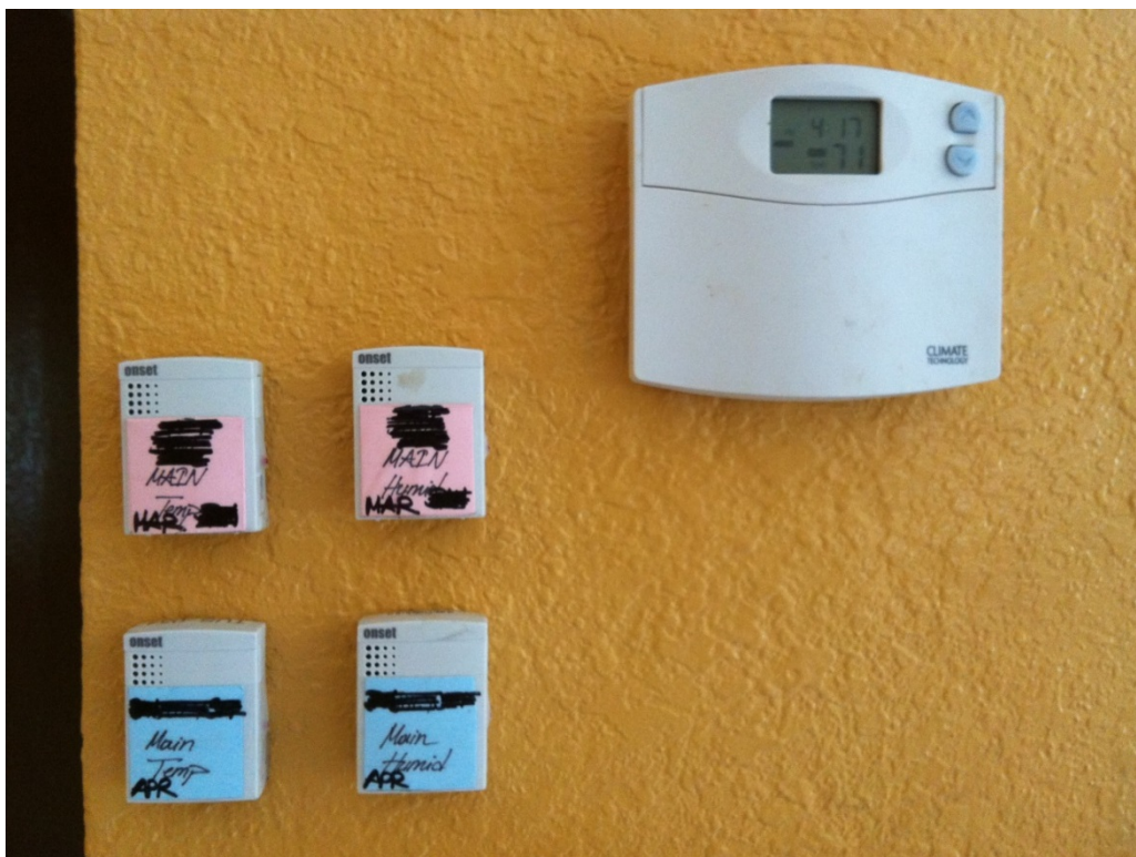
Figure 3-7 Inside temperature logger installed next to the current thermostat
