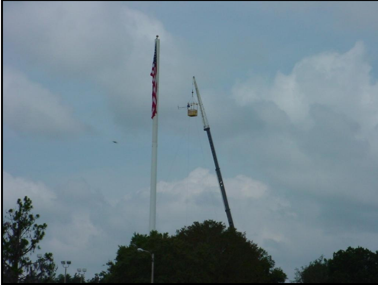
Figure 3. One of the crane mounts setup with transmitter for data collection.
