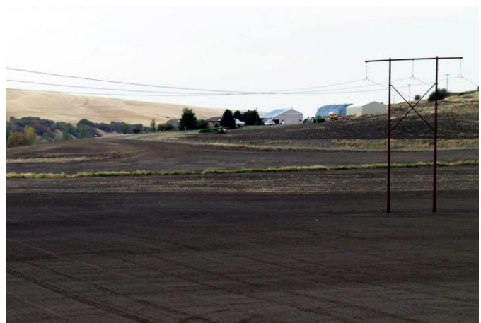
(b) span between pole 16/6 and 16/7
