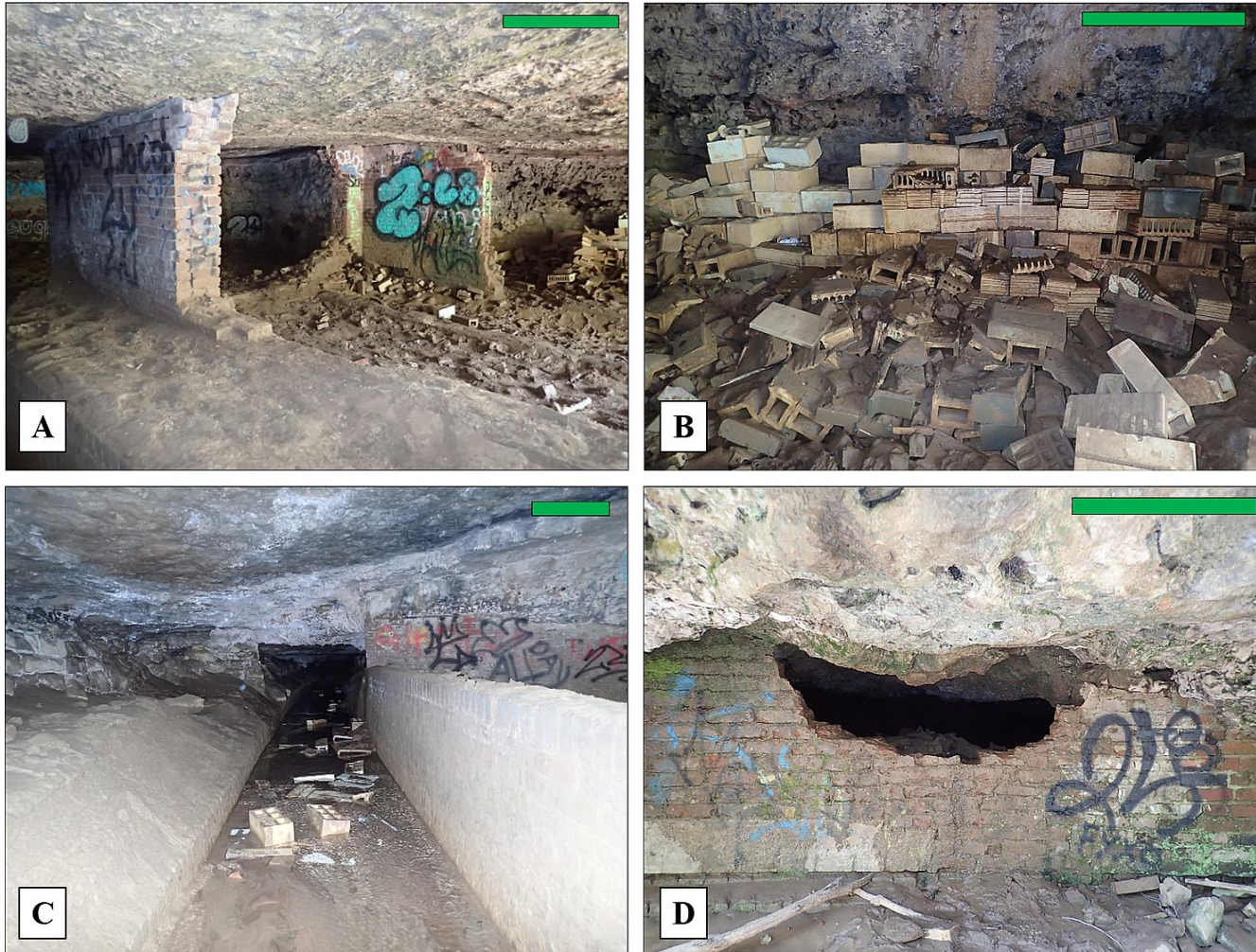
FIGURE 4. Brickwork and passages in Sauerkraut Cave. A , B , and C . The brick walls, block pile, and brick trough channelizing the stream in the front chamber of the main passage. D . Entrance to the side passage. Scale bars = 1 m. (Photographs by J. Gavin Bradley)
