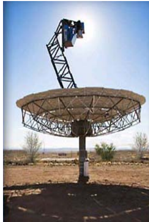
Figure 6: Suncatcher Solar Parabolic Dish Stirling Energy System by SES [64]
