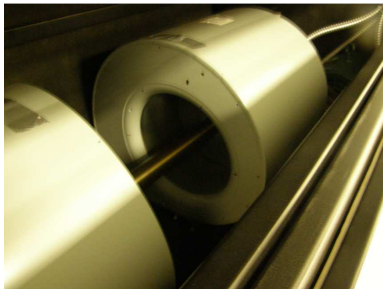
Figure A 23: Centrifugal fans within CRAC.
