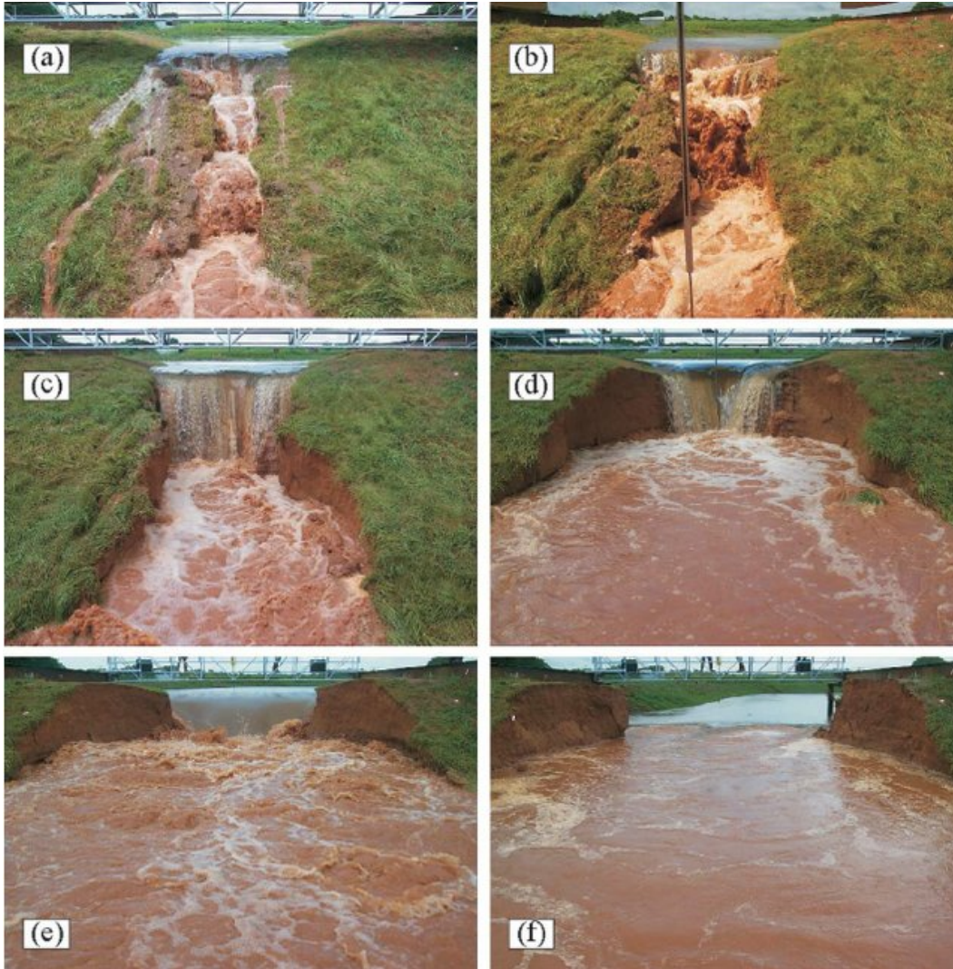
Figure 1-4: An illustration of the dam breaching process by overtopping: (a) rills and cascade of small overfalls at t = 1/4 7 min; (b) consolidation of small overfalls at t = 1/4 13 min; (c) headcut at downstream crest at t = 1/4 16 min; (d) headcut at upstream crest at t = 1/4 31 min; (e) flow through breach at t = 1/4 40 min; (f) transition to final breach stage at t = 1/4 51 min [14].
