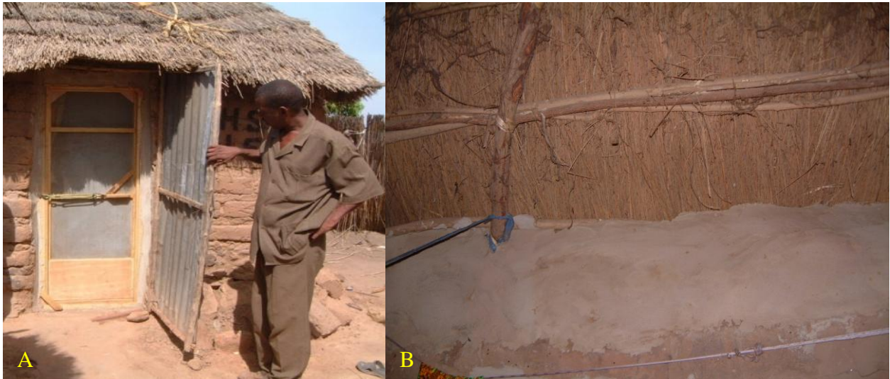
Fig. 2.1a) screened door, b) eaves closed with rubble and mortar
